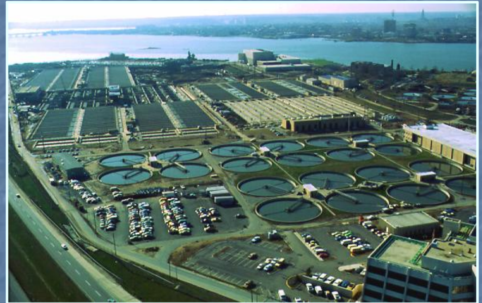
Blue Plains Wastewater Treatment Plant
